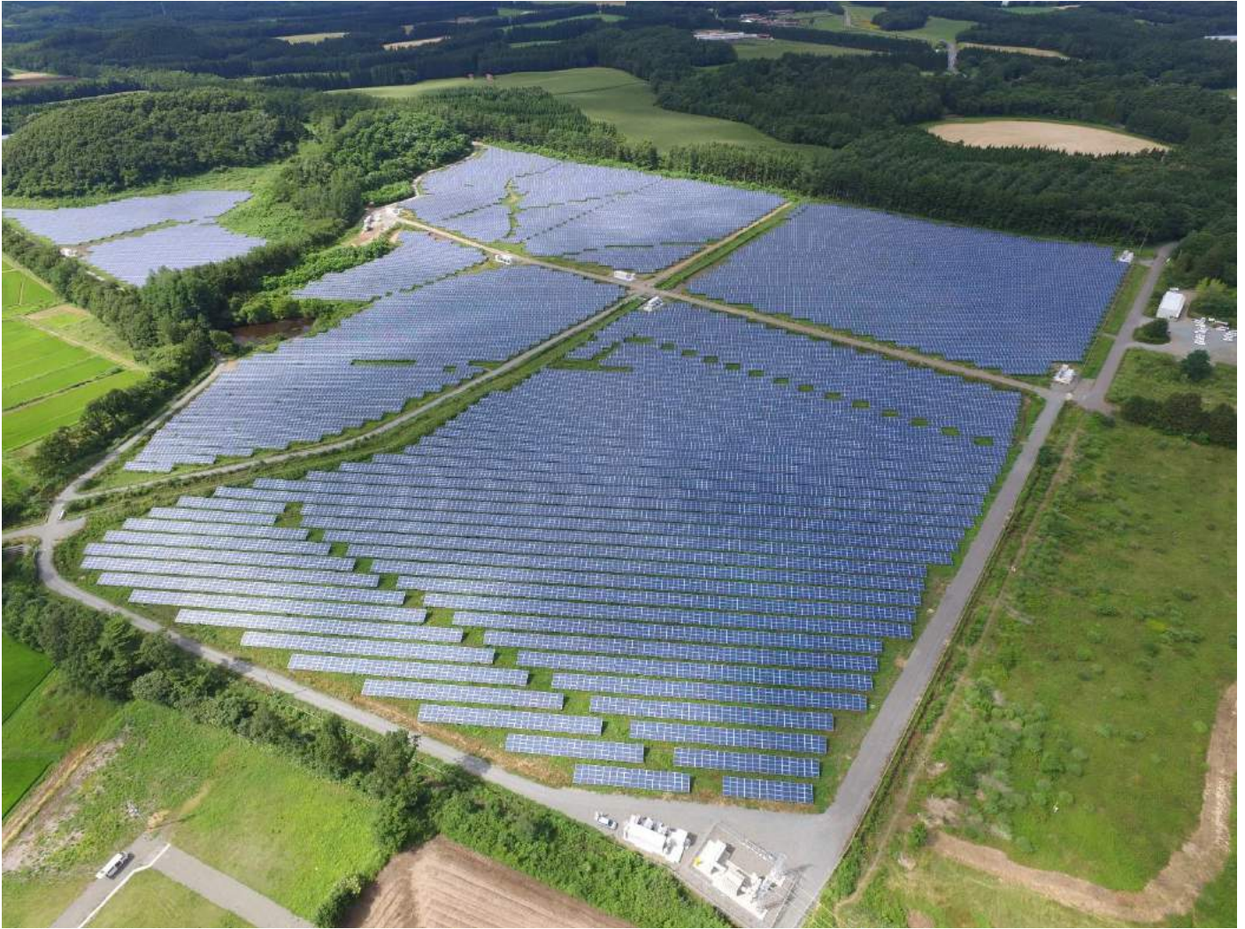
Shizukuishi solar power project in northern Japan
